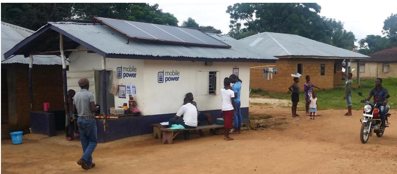
Photo: Mobile Power Hub for charging battery packs and acting as a focal point for local communities.
