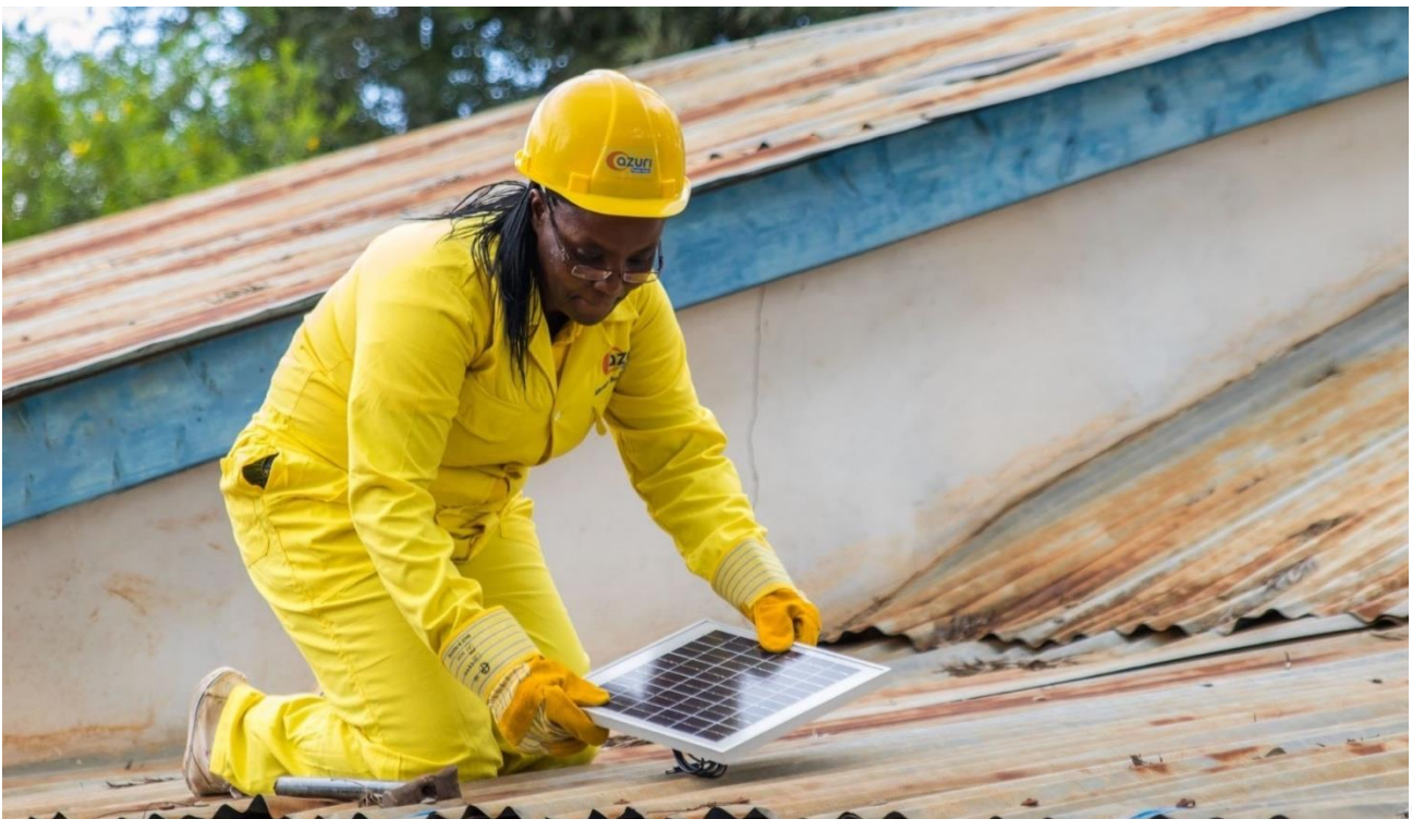
Photo: Azuri engineer installing a solar panel on a rooftop
